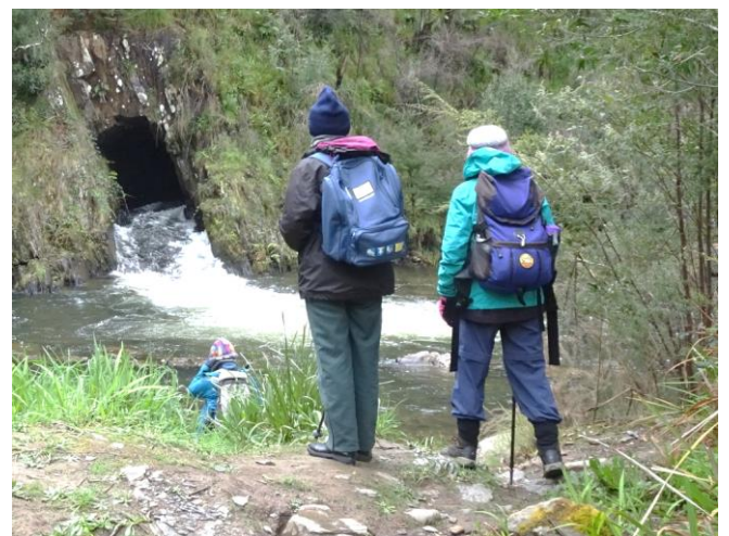
The outlet of the Horseshoe Bend Tunnel (Photo: Phil Rayment)
