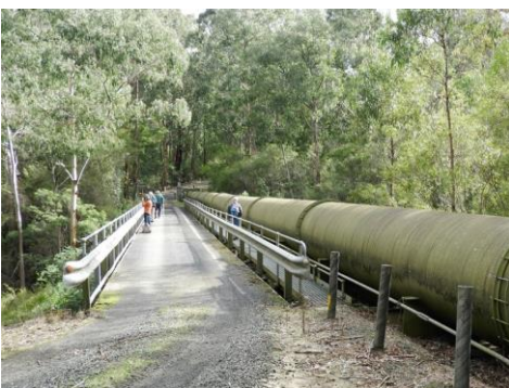
The pipe from Moondarra Reservoir (Photo: Irene Proebsting)
