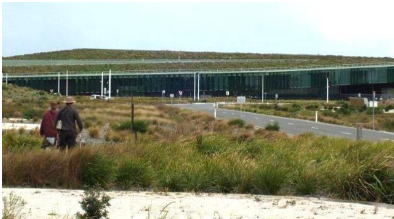
Vegetation growing on the roof of the building (Photo: Peter Ware)
